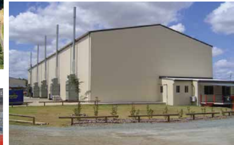
South Carolina USA Facility
