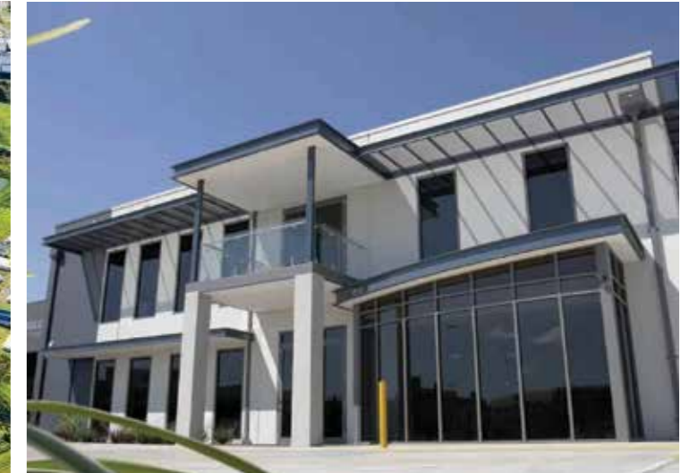
Forrestdale WA Facility
